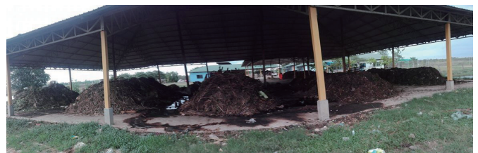
Figure 7: Composting Plant Operated by COMPED
