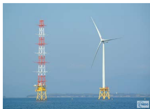
Wind power generation
