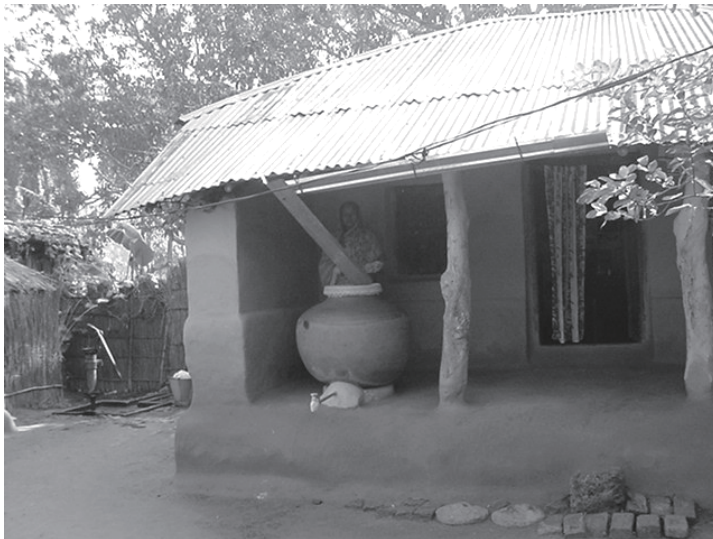
Figure 6. A rainwater harvesting system in a rural area of Bangladesh
