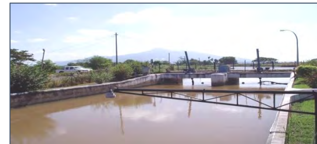
Regulator & Water Level Station
