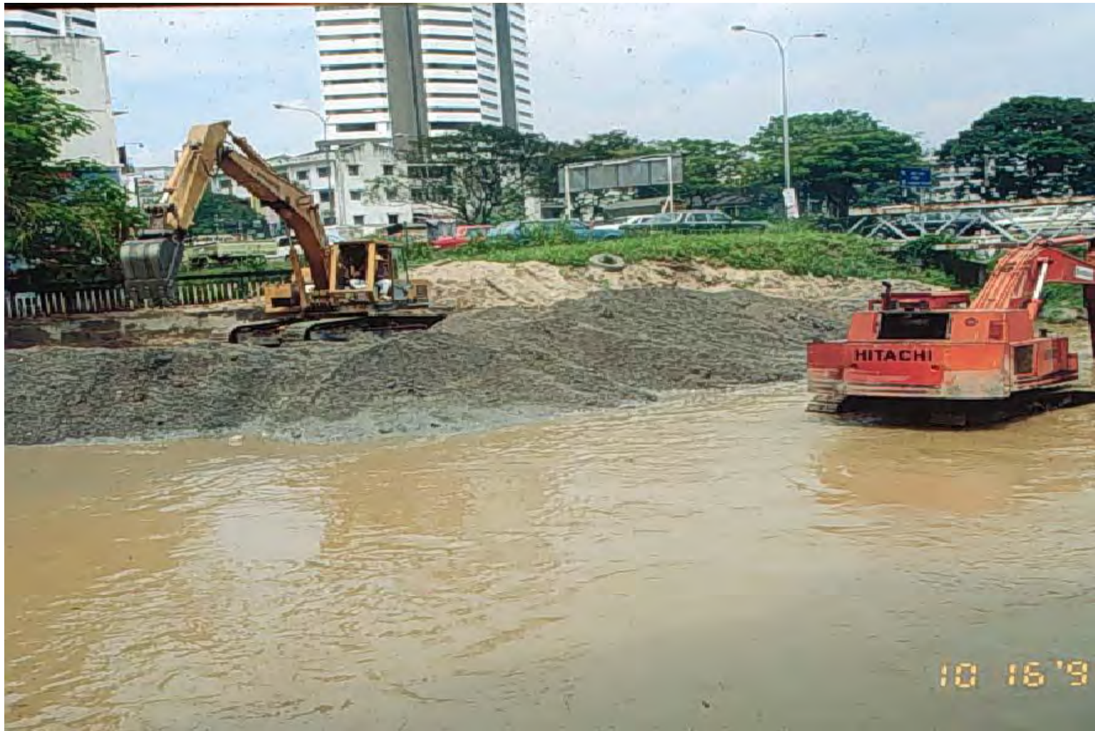
Widening of The River Channel
