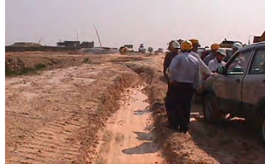
Erosion and Sediment Control
