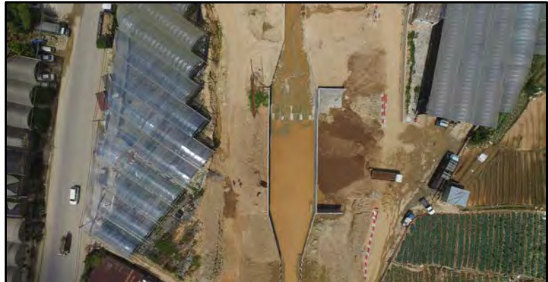
Drop Structure 4 - CH 1450
