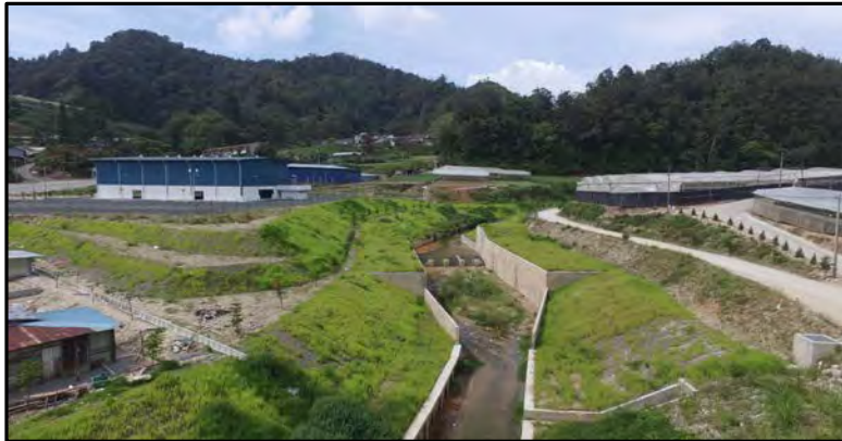
Drop Structure 3 - CH 300
