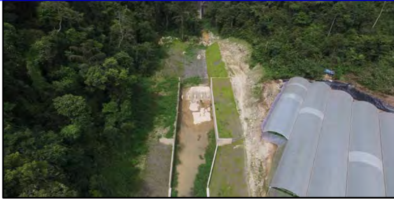
Drop Structure 1 - CH 100
