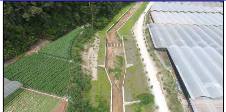
Drop Structure 2 - CH 200
