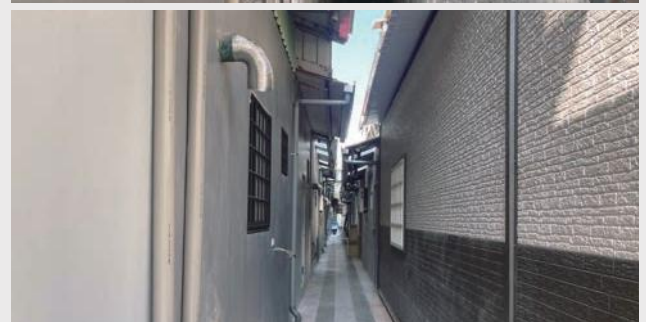
▲ Back alley before and after the construction of sewage pipes
