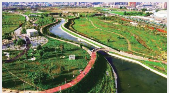
▲ The detention basins in Central Park with temporary rainwater storage and flood control functions.
