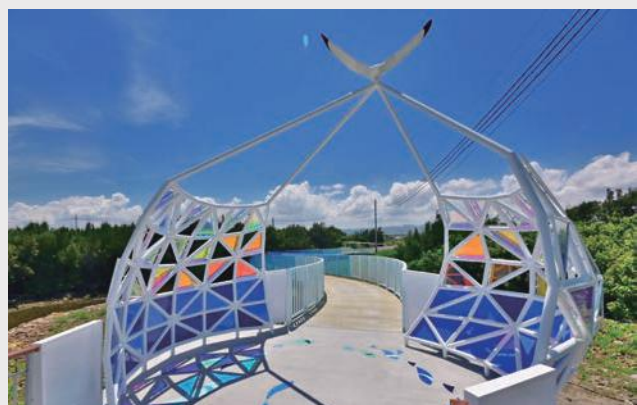
▲ Bicycle Path of Landscape Bridge at Songbai Fishing Port
