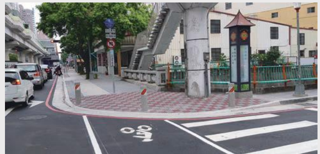
▲ Wenxin Road fan-shaped barrier-free ramp
