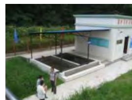
Facility for Sludge drying
