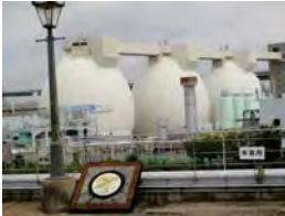
Higashinada sewage treatment plant
