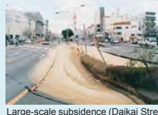
Large-scale subsidence (Daikai Street)
