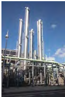
(1) Refining facilities 330 m 3 /hour, 2 systems (volume of digestion gas)
