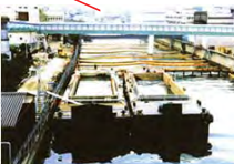
Sludge Thickening Facilities
