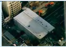
Building collapsed over road (Flower Road)
