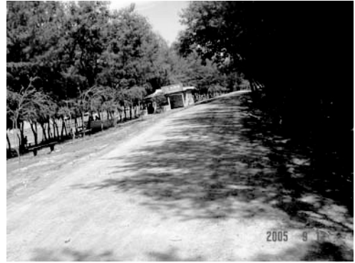
海岸堤防 (Patenga in Chittagong District with afforestations)
