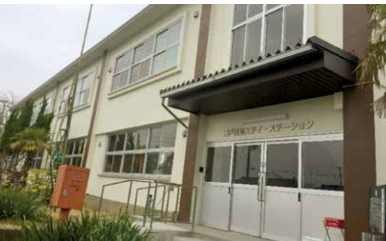
Figure 5. Stay Station: The building was previously an elementary school and was used as the main evacuation center following the tsunami in 2011 (Photo: Akane Minohara)
