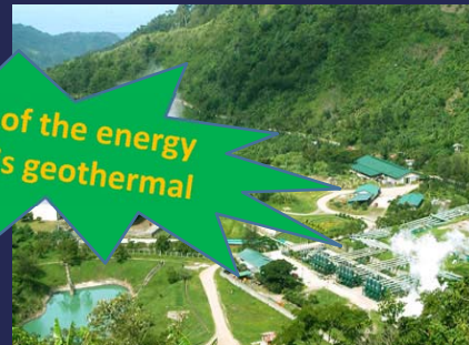
Palinpinon Geothermal plant
