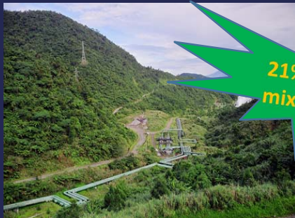
Bacman Geothermal plant
