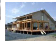
Higashida Eco House
