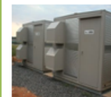
← Capacitor (Stabilizer of power variation in wind power generation systems)
