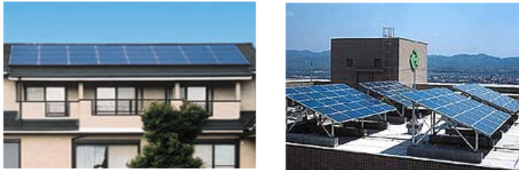
Photo Voltaic System (left: residential, right: commercial)
