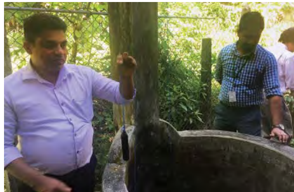
Figure 4.3.2. Installation of well data logger
