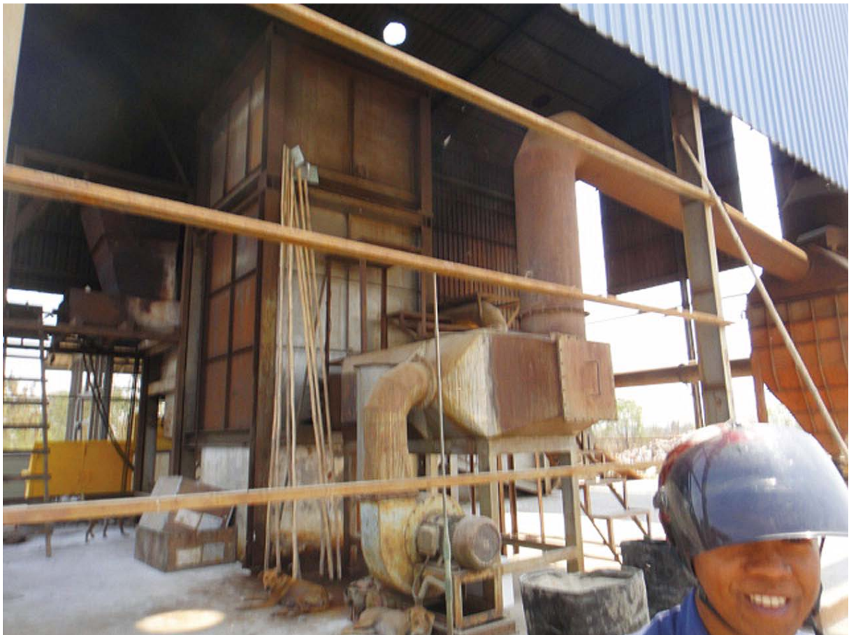
Figure 11: Incinerator stopped in operation. Source: IGES, 2016
