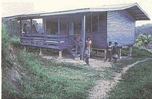
Model house constructed of certified timber - PNG
