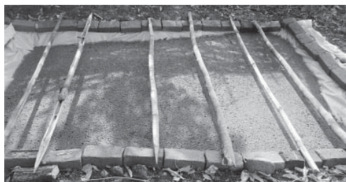
Construction of an Azolla Pit as a green fodder supplement for cattle feeding
