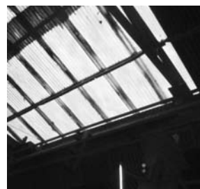
Translucent sheets for day light in workplace
