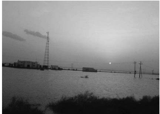
Flooded power station (Copyright: Author)
