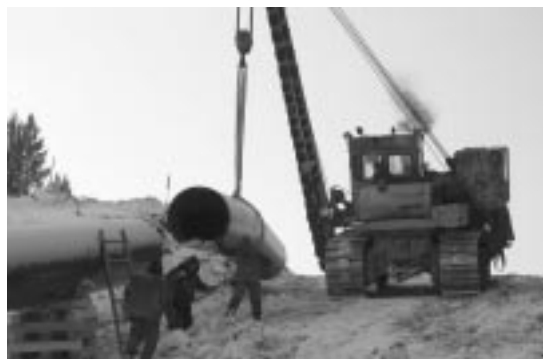
Pipeline construction on the Northern Amurskaya Oblast (Tynda District) Photo by Tatiana Tonkikh (Tynda)
