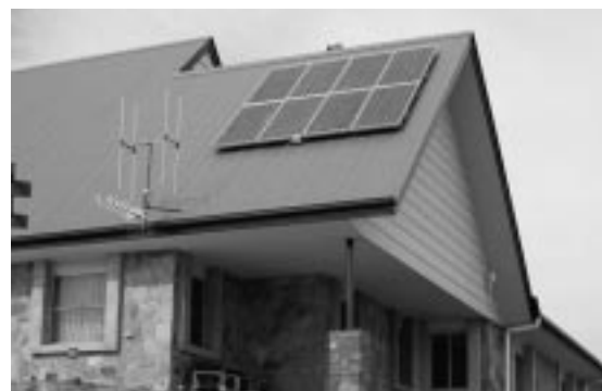
Solar panels ©DEWHA
