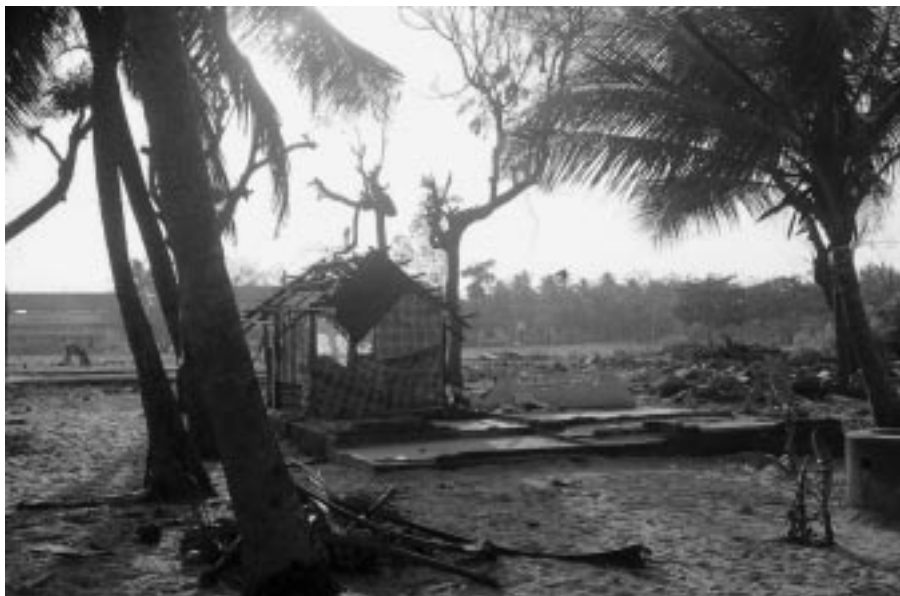
The tsunami damaged coastal houses and lands
