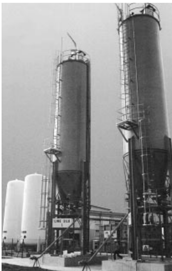
The Tuas desalination plant, the first for Singapore and the Asia-Pacific
