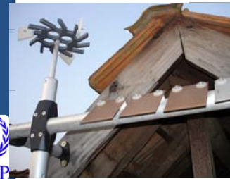
Corrosion monitoring track installed in Kathmandu, Nepal
