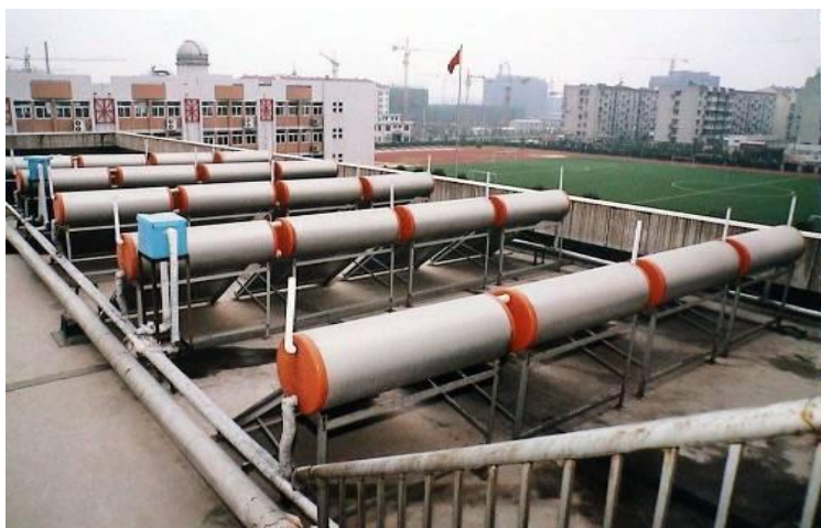
Roof solar heater in the affiliated high school of the Jiangsu
