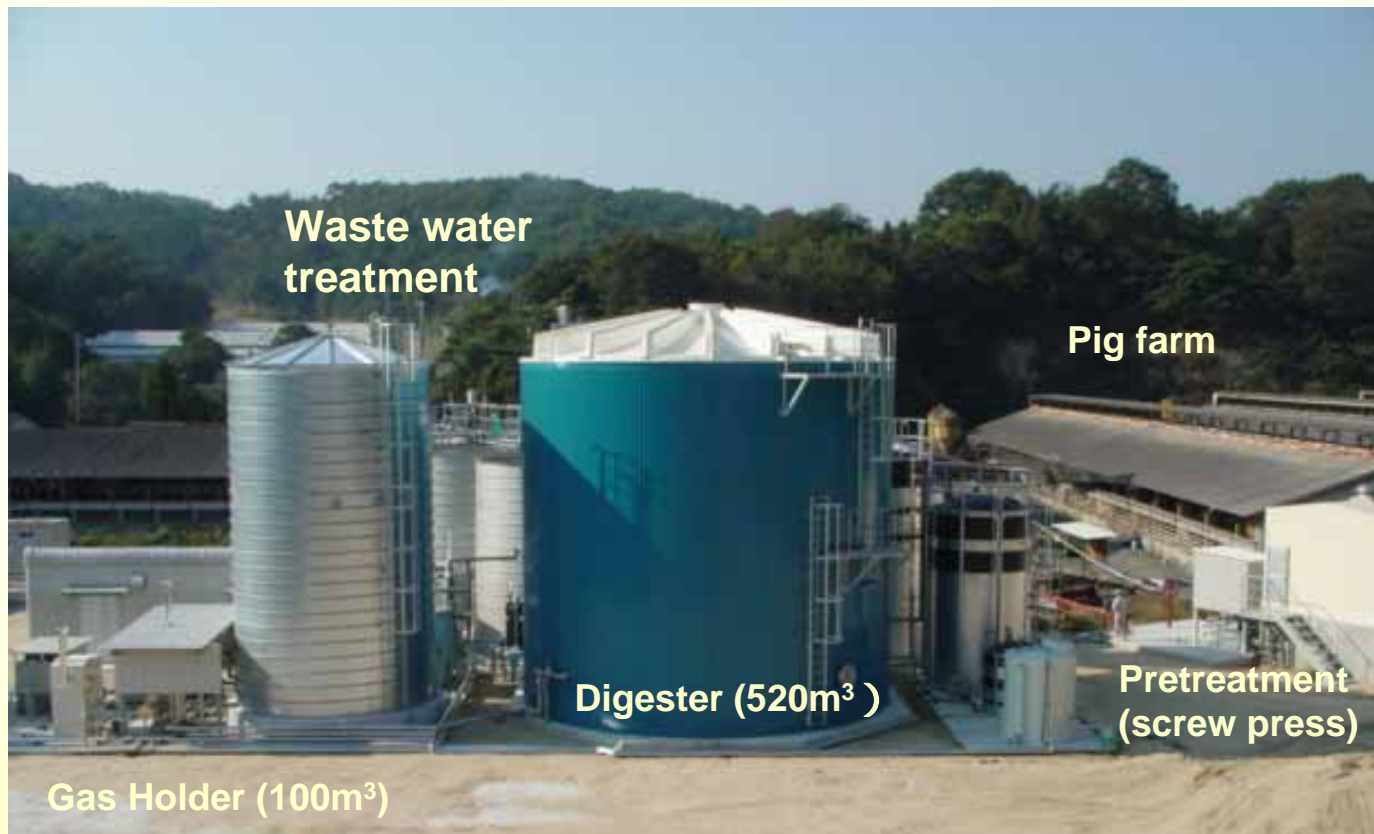
Pilot plant in Hiroshima for Swine manure treatment
