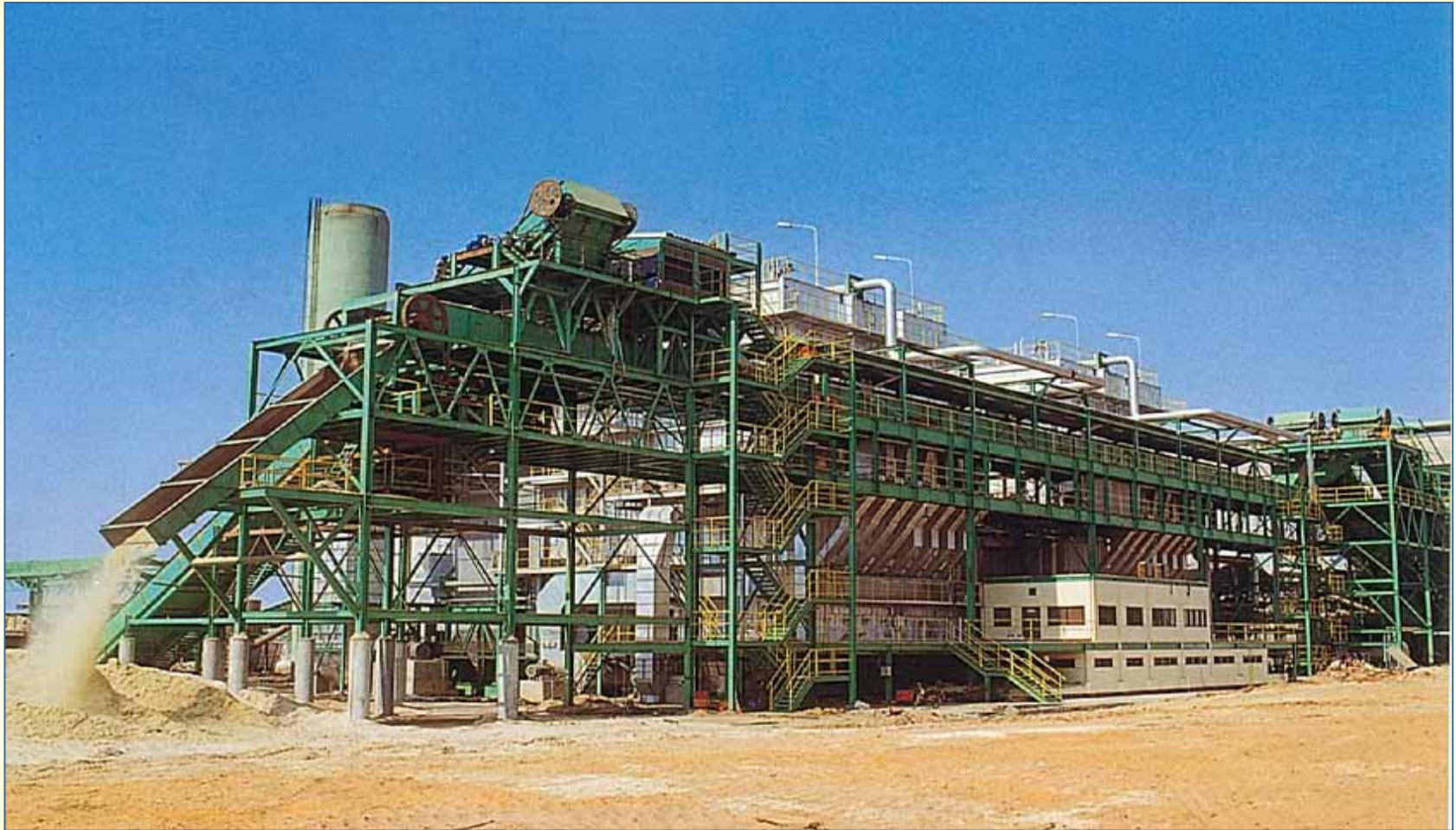
A bagasse firing boiler in a sugar factory of Thailand (300t/h 2units).
