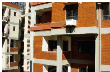
T-Zed apartment blocks showing projecting and receding massing creating shading for the lower floors
