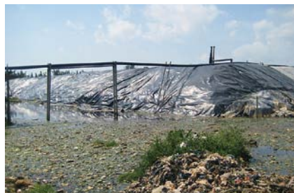
Methane transport pipes in Pontianak
