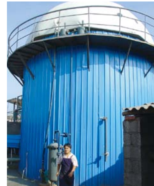
200m 3 integrated biogas plant for animal waste treatment in Badaoshao
