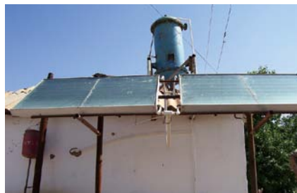
Solar-thermo Panel Installation (exterior, shower premise, School Bahardock)
