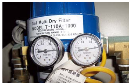
Installation the pressure gauge to measure loss at Multi Dry Filter
