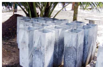
Biosand filter being constructed
