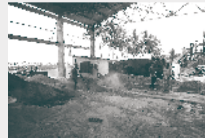
Biomass utilisation facility in southern part of India
